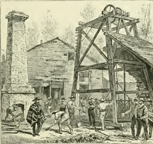
Coal Shaft, Arauco Railway Coal-Field.
