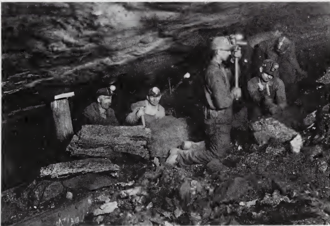
Anthracite miners in eastern Pennsylvania still used the pick, shovel, and hammer when this photograph was taken in 1930. Although the United Mine Workers of America would soon reorganize these coal fields and challenge the power of the Philadelphia-based railroads that owned these mines, the union could not forestall the postwar decline of anthracite as a heating fuel and the subsequent impoverishment of the region. (Hagley Museum and Library)
