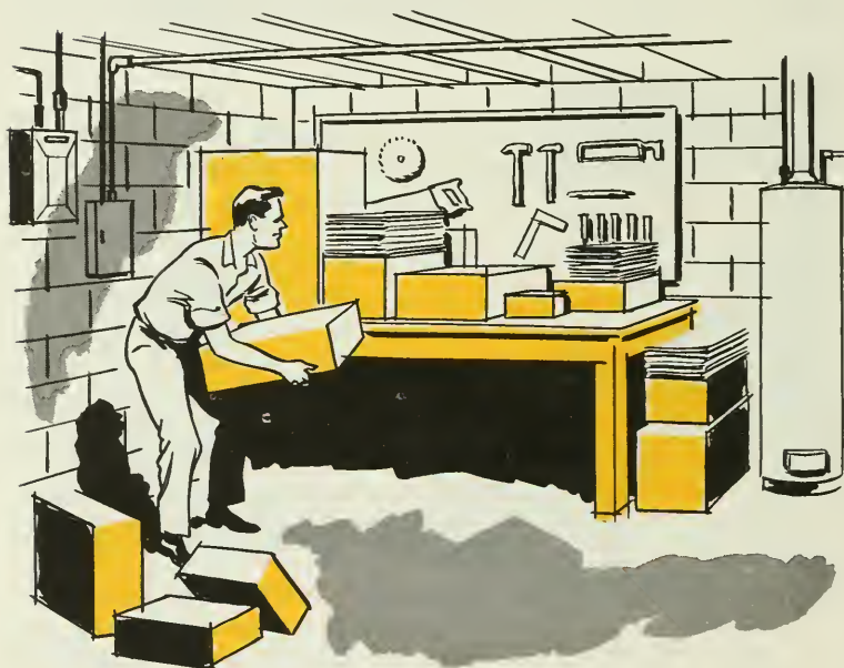
This man is improvising a fallout shelter in a basement corner by stacking heavy material on and at the open sides of a sturdy table. Piling dirt and other heavy material in the basement window wells will improve his margin of protection.
