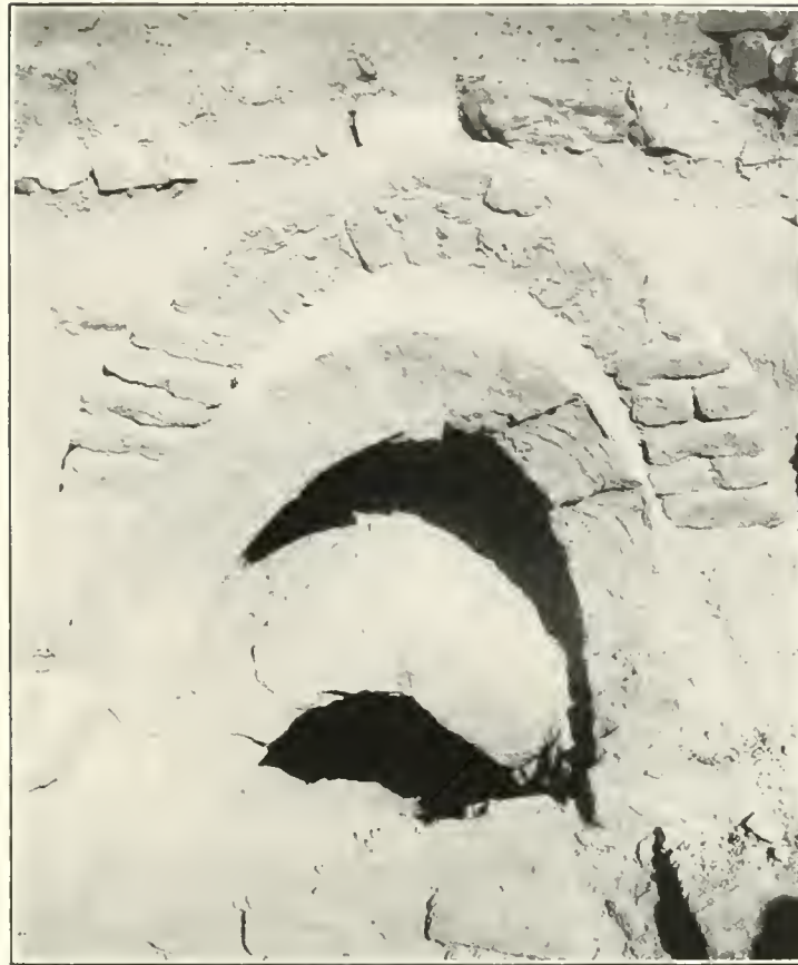
(a) View of Tomb 38, showing the brick vaulting
