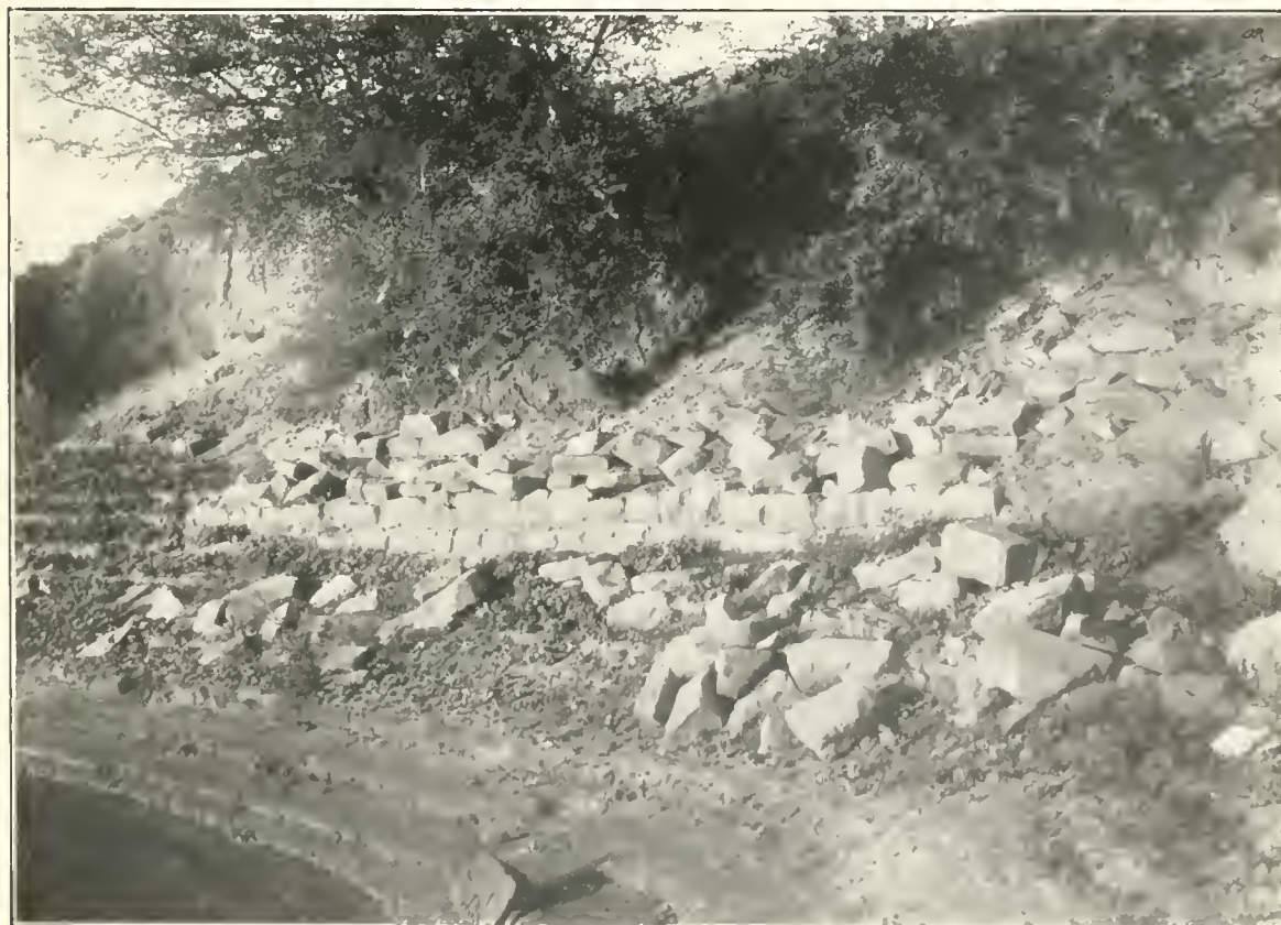
(b) Stone retaining wall on the river front at Shablul
